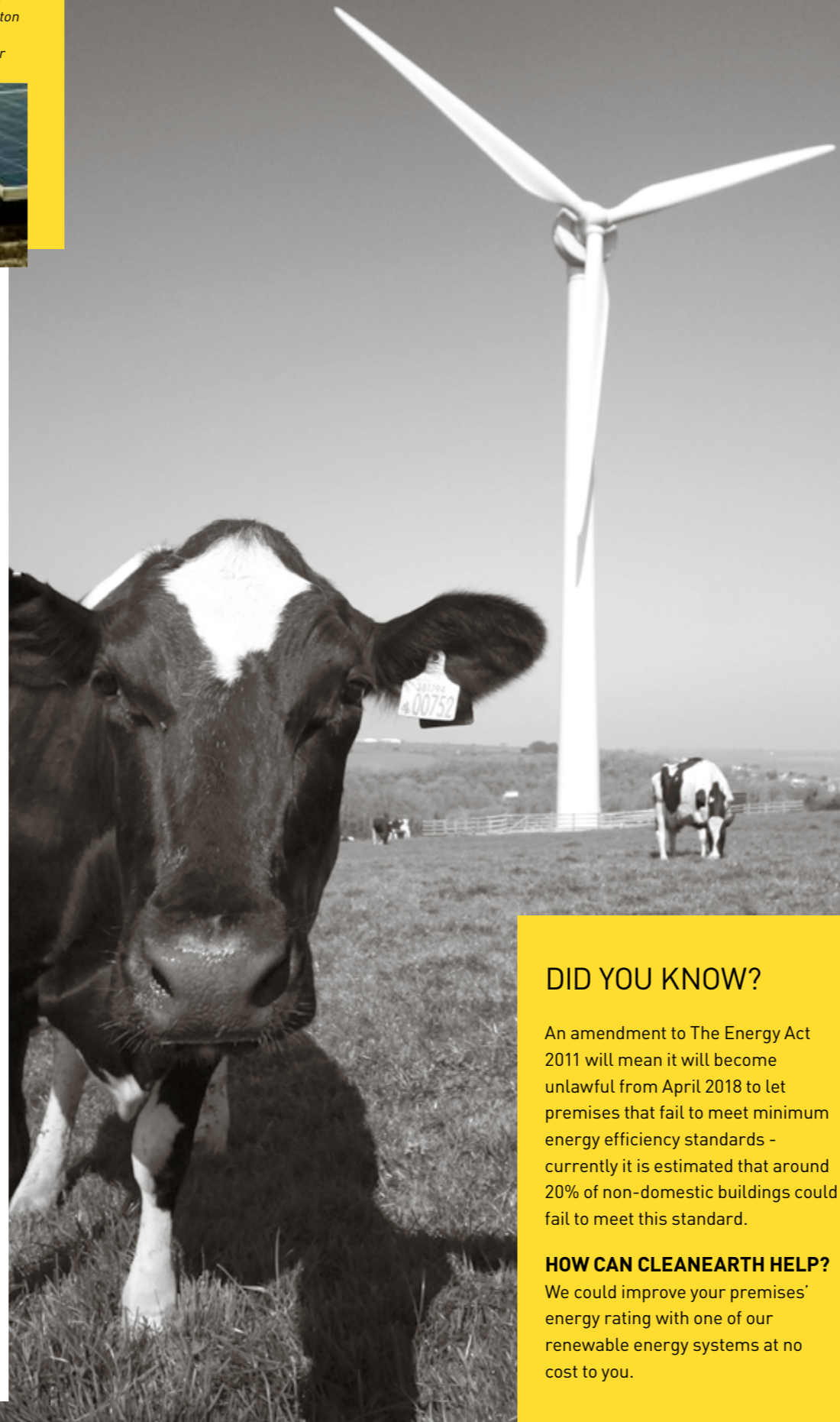
CleanEarth 500kWp turbine installation at Pengelly Farm (see page 7 for more information)
