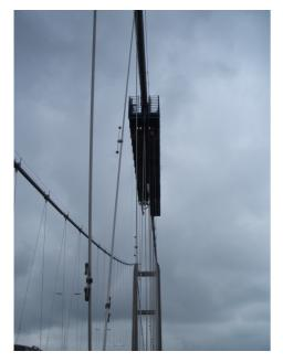
Once ALPS had carried out the lift the man working platform was secured in place and a powered feeder cradle was installed to ensure operatives and equipment could be transported vertically too & from the working platform.
