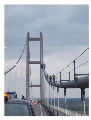
Above: The main cable access platform is installed by ALPS specialist Rope Access operatives using 4 x 3000Kg rope conveying winches and safety devises; right >
