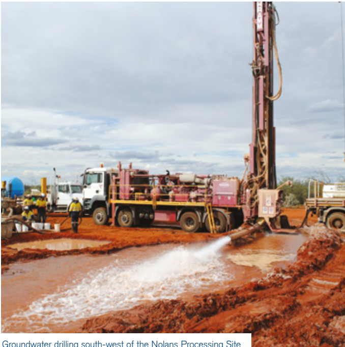
Groundwater drilling south-west of the Nolans Processing Site
