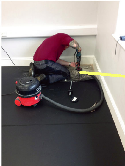
Drilling test holes (for % moisture) between underfloor heating pipes under rubber floor
