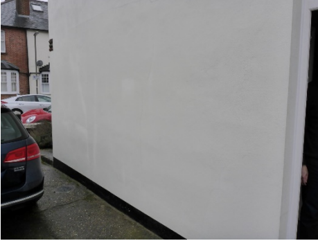
Render applied to the flank wall
