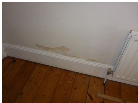
Saturation and damage at low level in the lounge
