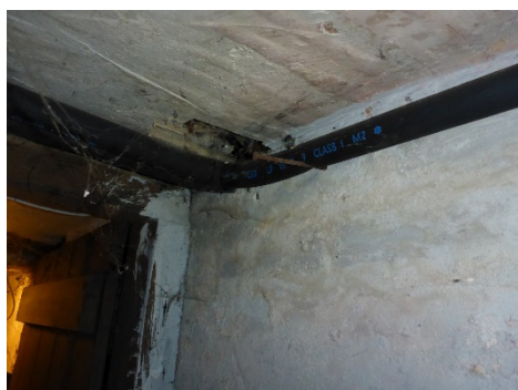
Signs of moisture penetration on the cellar walls
