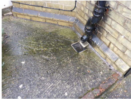
Rainwater discharge point to the front
