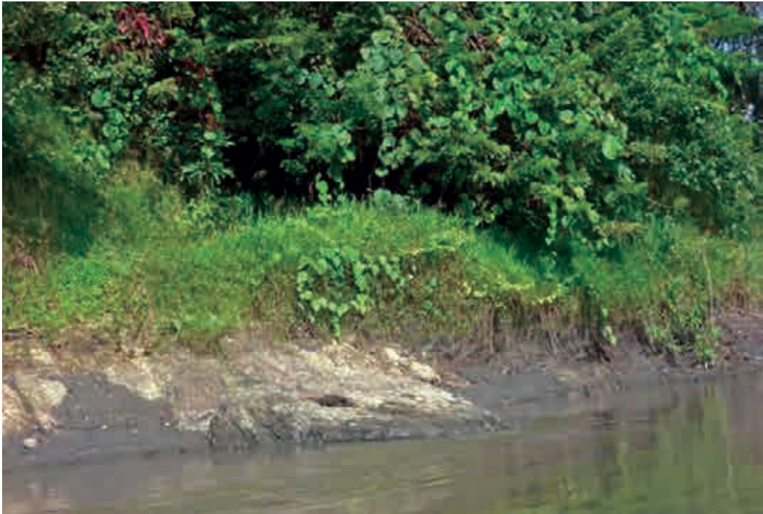
Figure 11. Bulldozer landing ramp
