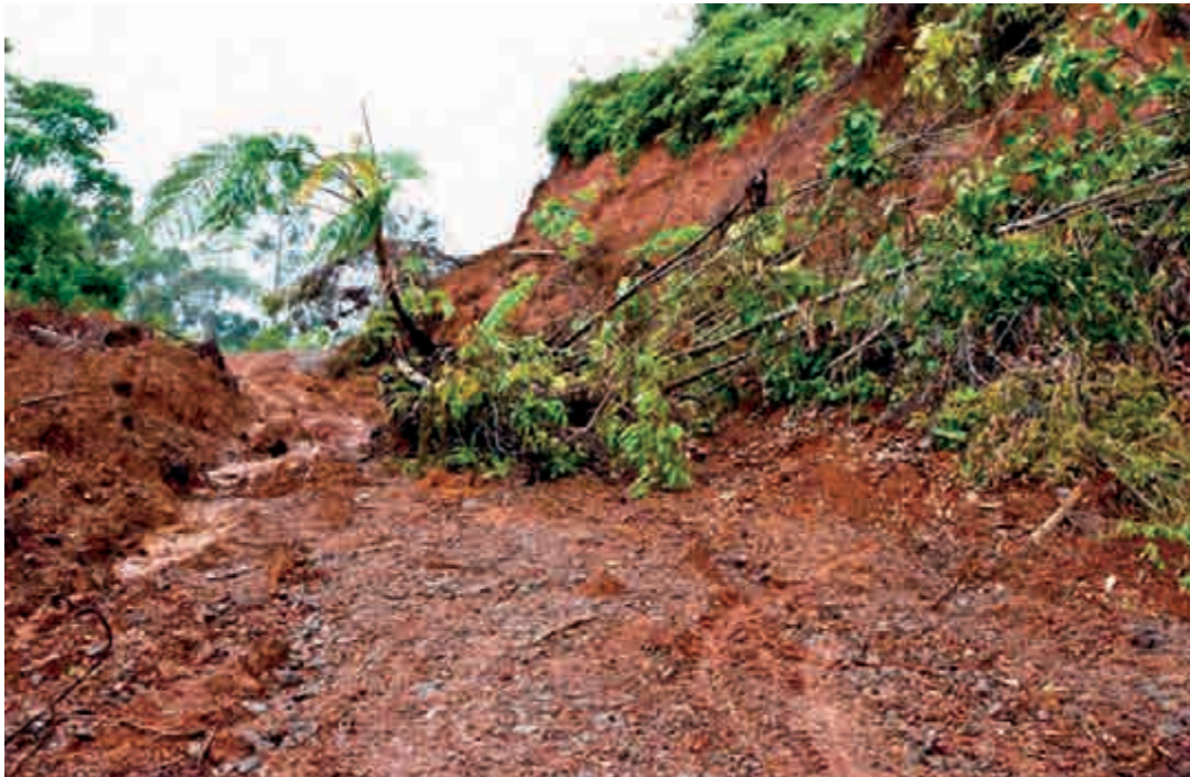
Figure 6. Road blocked by fallen tree
