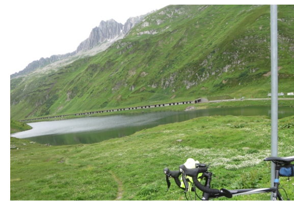
Last step: the avalanche tunnel
