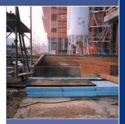
Regupol RAV200 prevented the transfer of road generated noise and vibration into a surrounding commercial development
