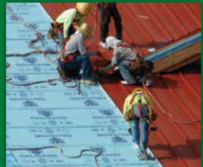
CUSTOM METAL ROOFING
