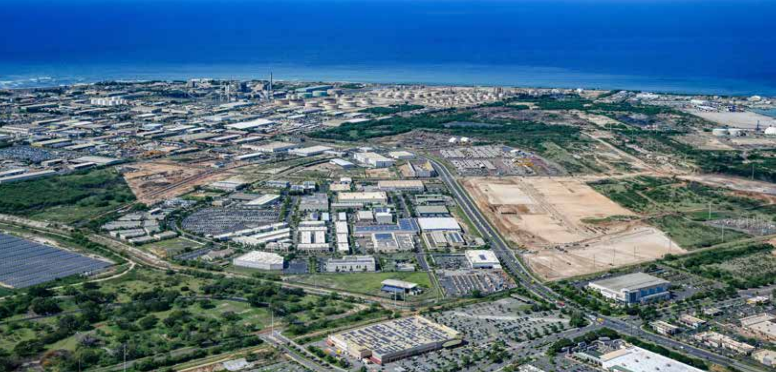
Avalon Development's 54-acre, industrial-zoned Kapolei Business Park West PHOTO COURTESY AVALON DEVELOPMENT
