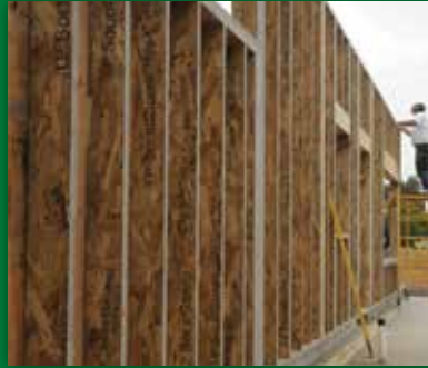
LSL WALL PANELS @ HOSPICE, KAMUELA
