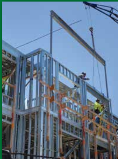
STEEL FRAMING @ KA MALANAI, KAILUA
