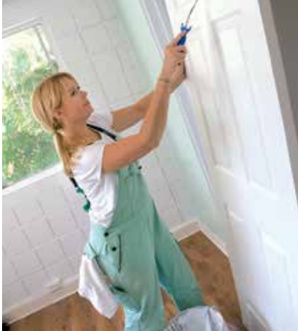
Hawaii renovator Angel Kay Uherek wears Rosies Workwear on the job.
