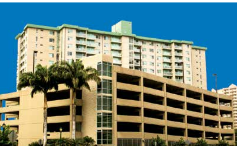
Country Club Village 6 in Salt Lake is one of the rare recent residential high-rise projects located outside Honolulu’s urban core. PHOTO COURTESY HAWAIIAN DREDGING CONSTRUCTION CO. INC.
