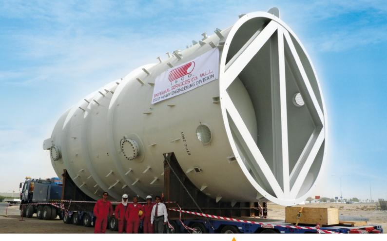
Equate Oilfien II EBSM, Shuaiba L 15m x W 6.7m x H 8.1m G.Wt.110 Ton Delivery Location: Shuaiba Equate. Crossed over busy traffic through Mina Abdullah-Shuaiba Refinery and transported to site.
