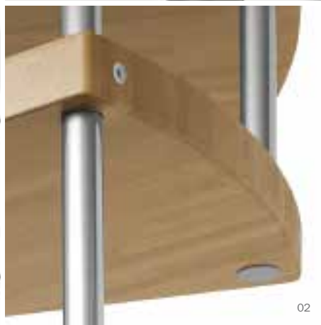
02 _ Baluster fixing to the tread.
