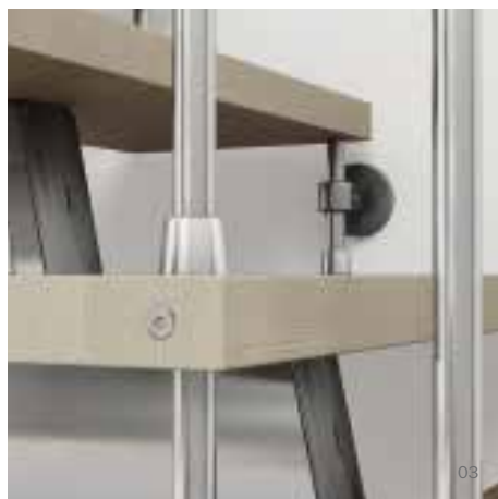
03 _ Baluster fixing to the tread.
