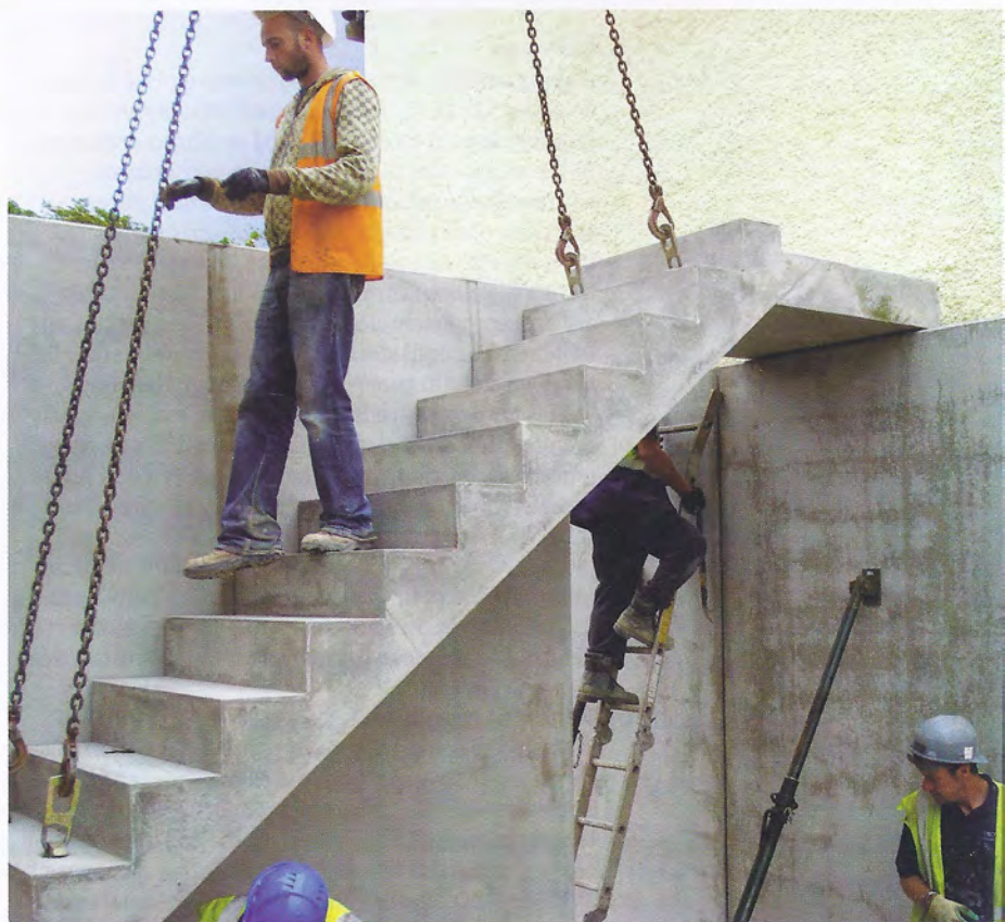
Above: Precast stair installation.
