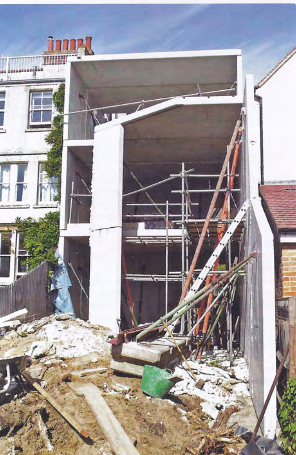
Above: View from rear during construction showing the concrete frame.
