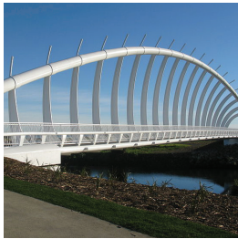
Waiwhakaiho Pedestrian Bridge
