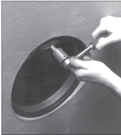
Install - Wedge Korbond with Socket Wrench & Torque Limiter
