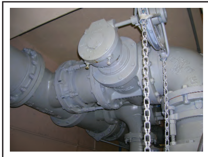
Cam-Centric® Plug Valve with worm gear actuator and chainwheel
