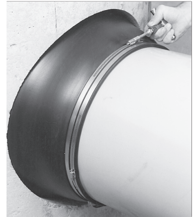
Install Pipe Clamp(s) with T-Handle Torque Wrench
