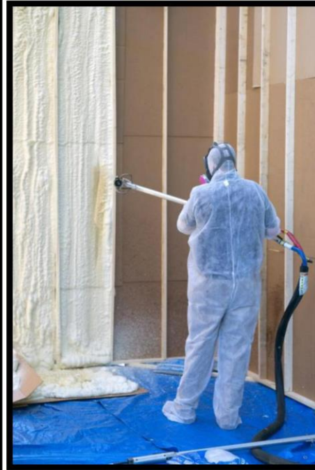
21-23 SEPTEMBER 2016. ON-SITE FOAMING DEMONSTRATION OF POLYMAC'S NEW SPRAY GUN EXTENSION HANDLES, WHICH ALLOW EASIER TREATMENT OF LARGE, HIGH WALL SURFACES.
