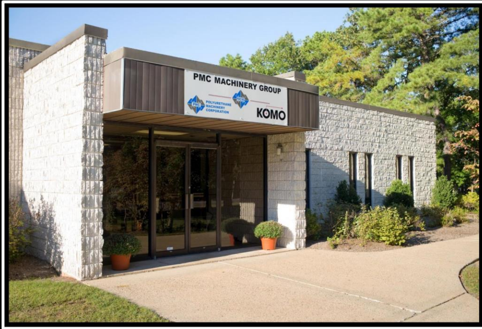
...AND RENOVATED BUILDING EXTERIOR WITH NEW SIGNAGE.
