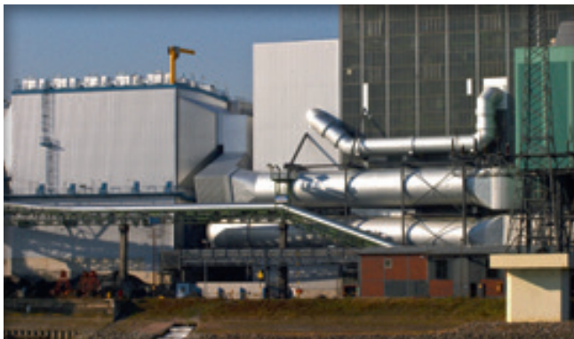
GKM GrossKraftwerk (coal-fired power plant) Mannheim, Germany
