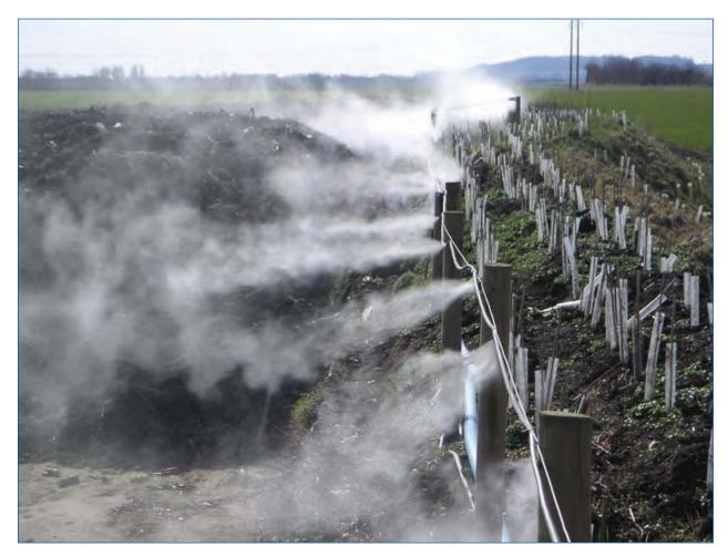
The Pacific 320 is a high-pressure water based system and is specifically designed to overcome odour emissions from widespread areas. The system forces water and *Odr 3*, neutralising agent through nozzle line often located along the site boundary. The resultant atomised mist acts as an effective barrier to control the odour emission.
