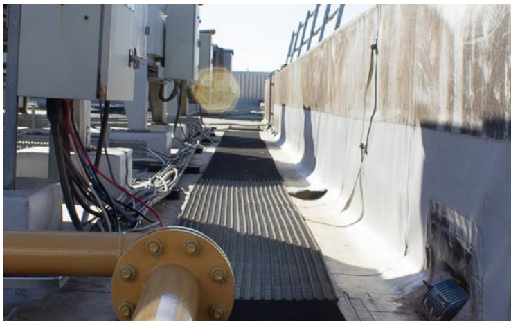
Left, Top: View of newly installed single ply around existing plant.
