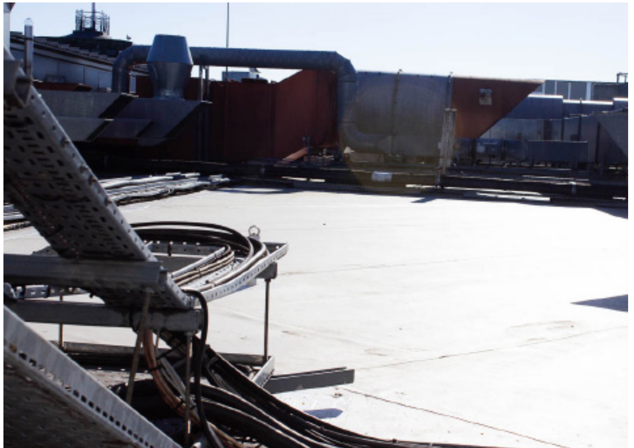
Left, Top: View of newly installed single ply around existing plant.
