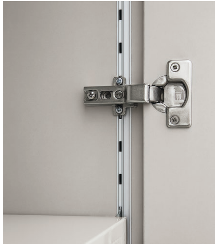
Hinged door on a metal rack
