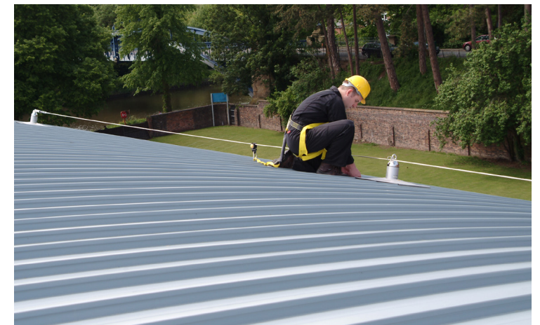
above : Mansafe system installed into single ply membrane
