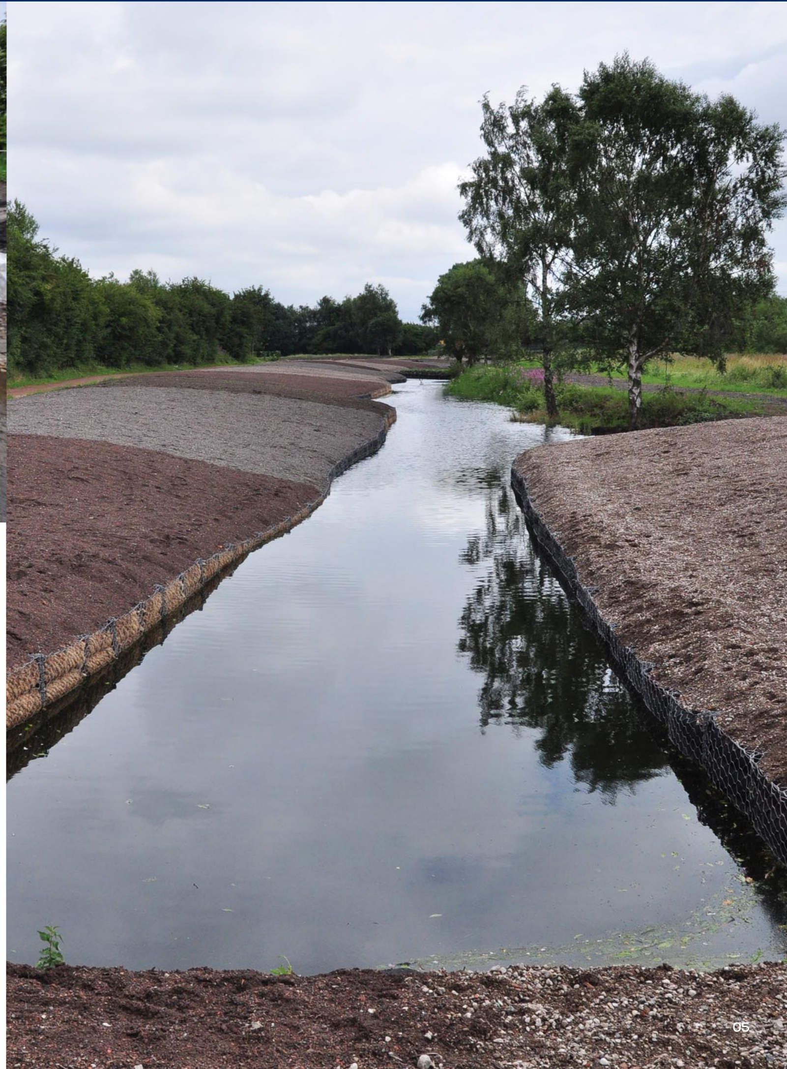
WOOLSTON CANAL CELTIC REMEDIATED CONTAMINATED SEDIMENTS WITHIN A CANAL BASIN AND USED THE TREATED SOILS TO CONSTRUCT A NEW LANDFORM ENCLOSED WITHIN GABION WALLS AND REED BEDS.
