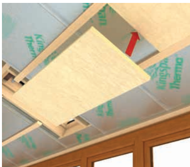
install insulation between batten.
