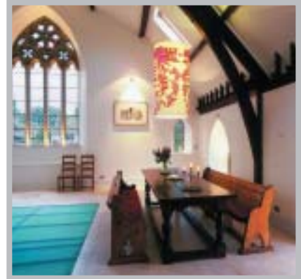
The new upper floor provides open plan kitchen, dining and living space. The opaque glass floor panels act as a light box when illuminated from below.
