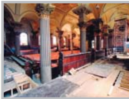
The church building viewed from gallery level during the restoration works.
