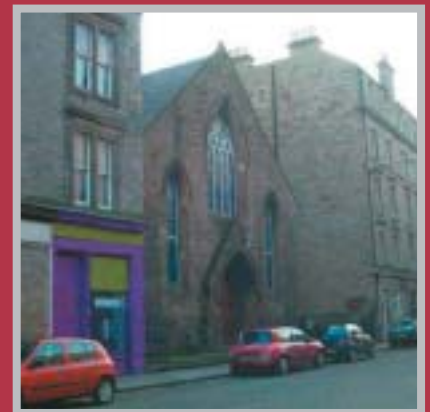
The former church building on Duke Street, now demolished.
