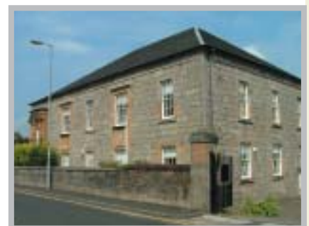
Simple classical 'box' style churches, such as the former Gaelic Church, have accommodated residential conversion well. Large 12 pane Georgian windows offer fine views and room settings.
