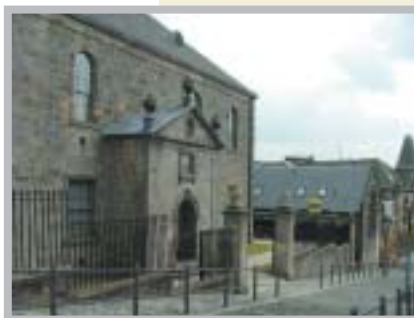
The elegant west elevation of the former Middle Church on Church Hill. The church last served as a place of worship in 1975.
