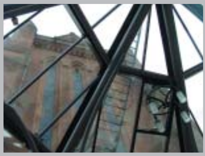
The Barony Hall Winter Garden is a glass roofed reception space created in the former courtyard between the Main Hall and the Bicentenary Hall.
