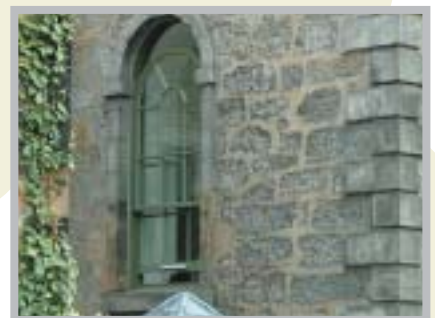
New timber sash and case windows on the former Middle Church are well designed and appropriate to the period of the original church building.
