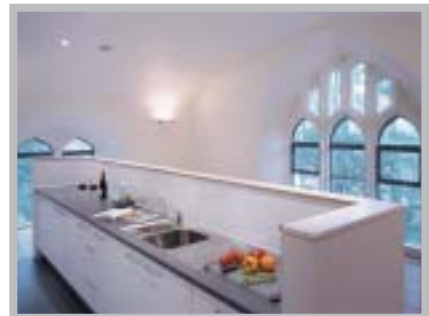
The original window openings played a key role in planning the conversion. New double glazed units improve the thermal value of the building whilst their low profile steel frame remains architecturally sympathetic.
