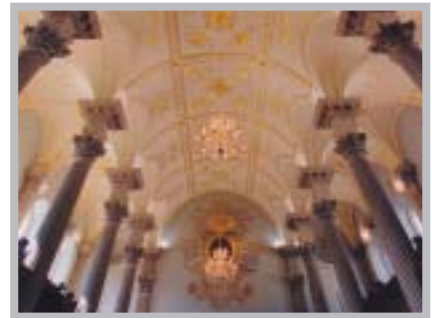
The main hall was returned to its original Georgian splendour. The ornate gilded plasterwork of the vaulted ceiling has been meticulously restored.
