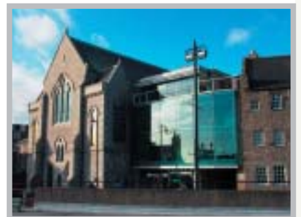
A new glazed intervention links the church building to the former Provost Ross's House, and clearly signals the museum's presence on Shiprow. Image copyright of Aberdeen City Council.
