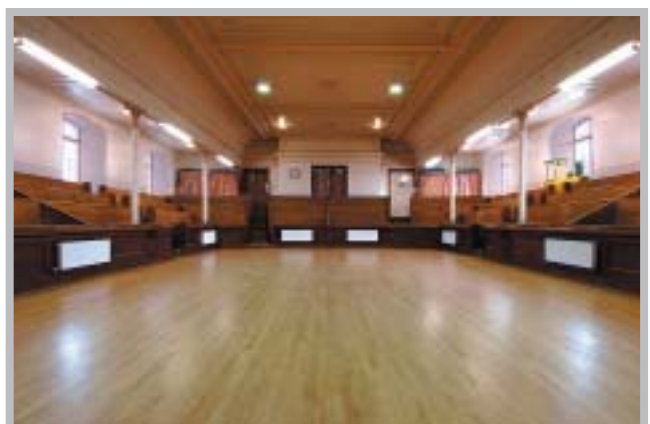
The space of the former church is well utilised: a new floor inserted at the gallery level has created the principal Arena Studio with the original pews retained to provide spectator seating. Copyright Dansarena Studios.
