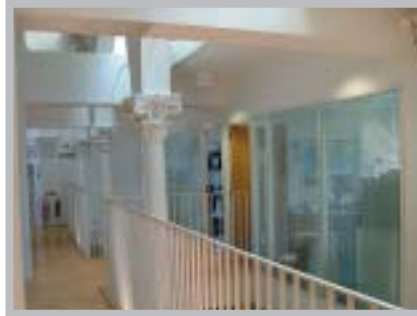
The original cast iron columns and architectural detail of the building add character to the circulation space and adjacent offices
