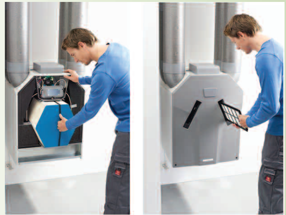
Cleaning the heat exchanger
