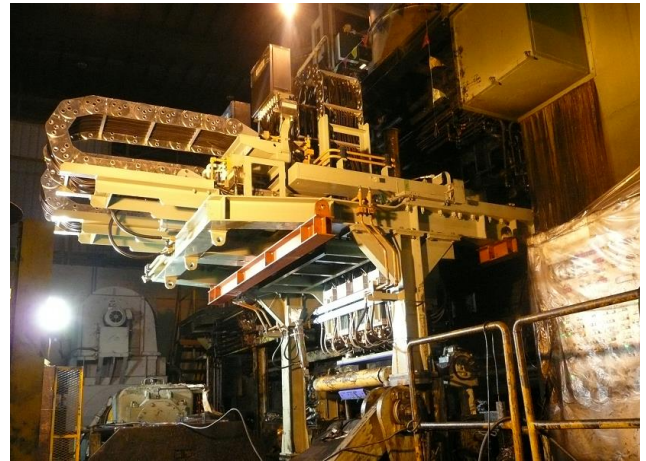
Figure 12. Zoom device in erection
