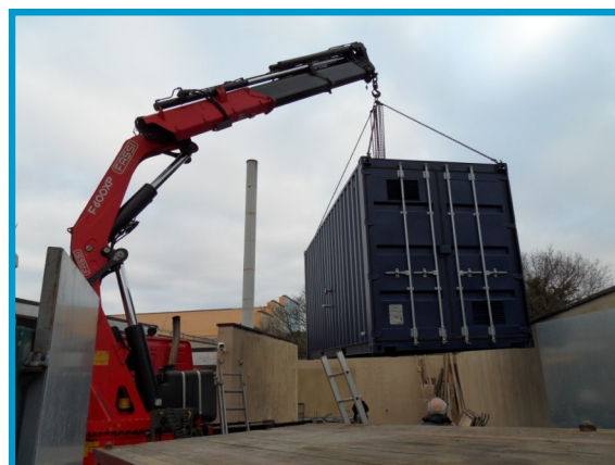
New boiler is craned into Pool yard
