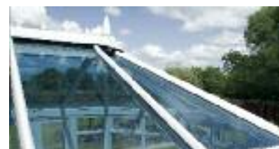
Glass units - reduce solar gain in summer and minimise heat loss in winter with treated glass.
