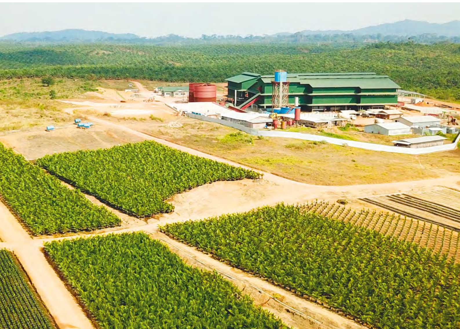
The new palm oil mill in construction at Palm Bay estate with part of the nursery in the foreground
