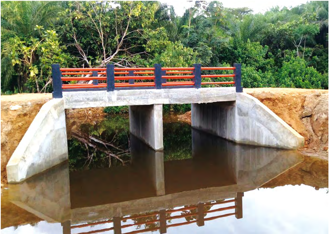
New concrete bridge replacing old wooden bridge at Robert Town
