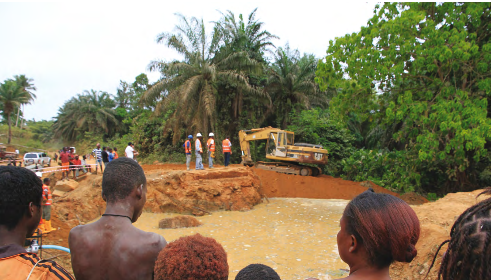
Construction of new bridge Palm Bay estate
