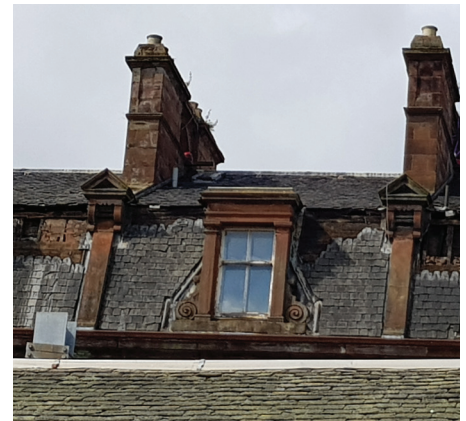
Station Hotel roof deterioration.
