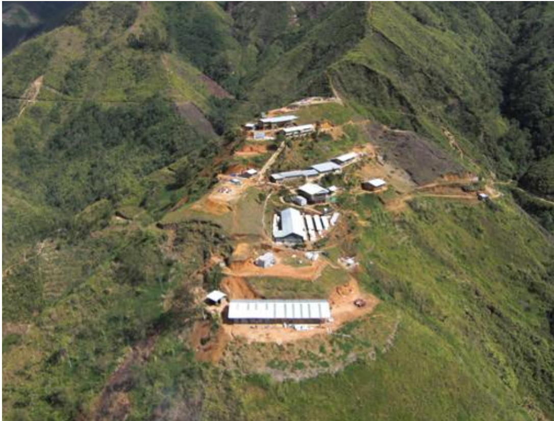
Figure 6 View of Current Site Infrastructure
