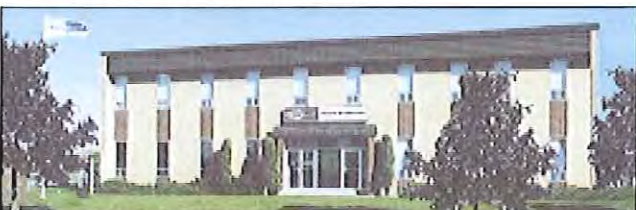
TORONTO, CANADA Velan-Proquip 41,000 sq. ft. (3,800 m 2 ) 2-48" (50-1200 mm) wafer check valves ½-24" (15-600 mm) clamp joint connectors, ISO 9001
