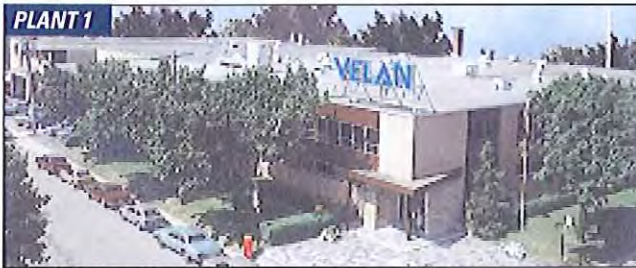
PLANT 1 MONTREAL, CANADA 109,000 sq. ft. (10,126 m 2 ) ¼-4" (8-100 mm) forged gate, globe & check valves, ASME 'N' stamp, ISO 9001
