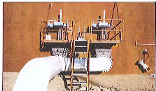
Cast steel valve installation at an oil refinery.
