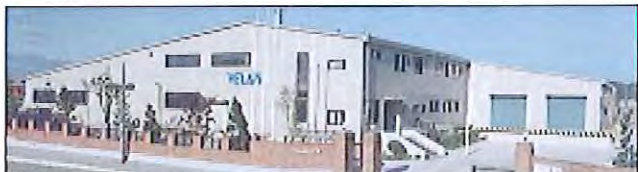
ANSAN CITY, SOUTH KOREA Plant 1 30,000 sq. ft. (2,800 m 2 ) components and 2-4" (50-100 mm) cast steel valves, ISO 9002
