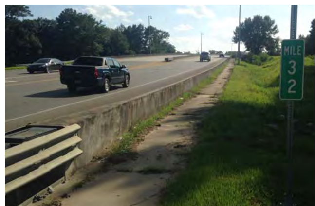
Existing sidewalk along Bay Bridge Road
