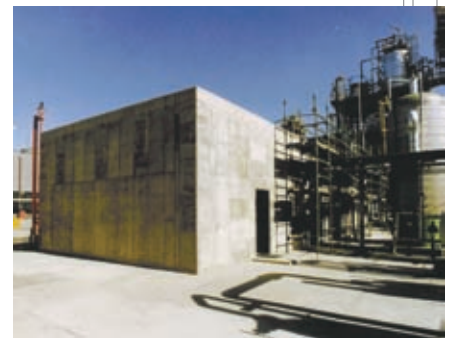
Blast Resistant Control Room under Construction
