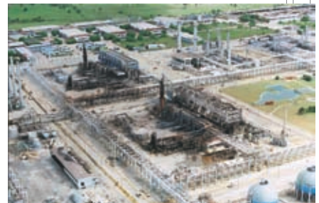
Gas Plant Vapour Cloud Explosion
