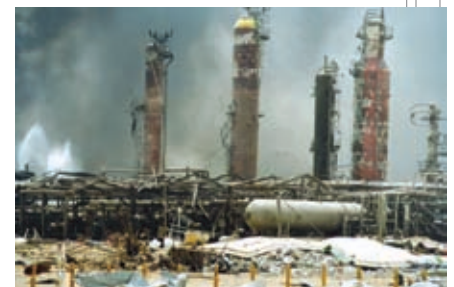
Aftermath of Accidental Vapour Cloud Explosion
