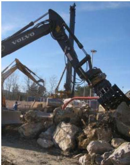
Grab BG16 on works of stone laying (making the scarps)
