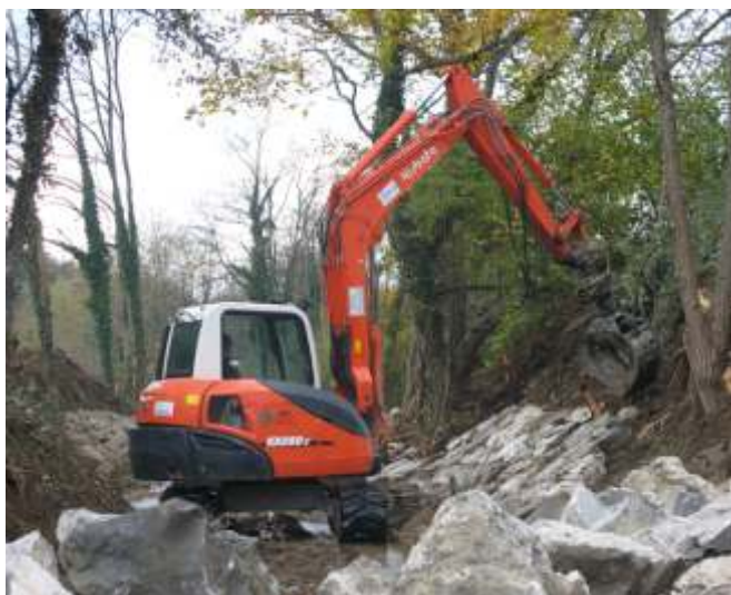
Using Grab BG8 for stone laying (making the scarps)
