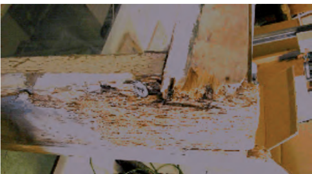
Top: Exterior view of test window as received; left detail showing the decayed sill; right detail showing the gap between the upper sash and the frame
