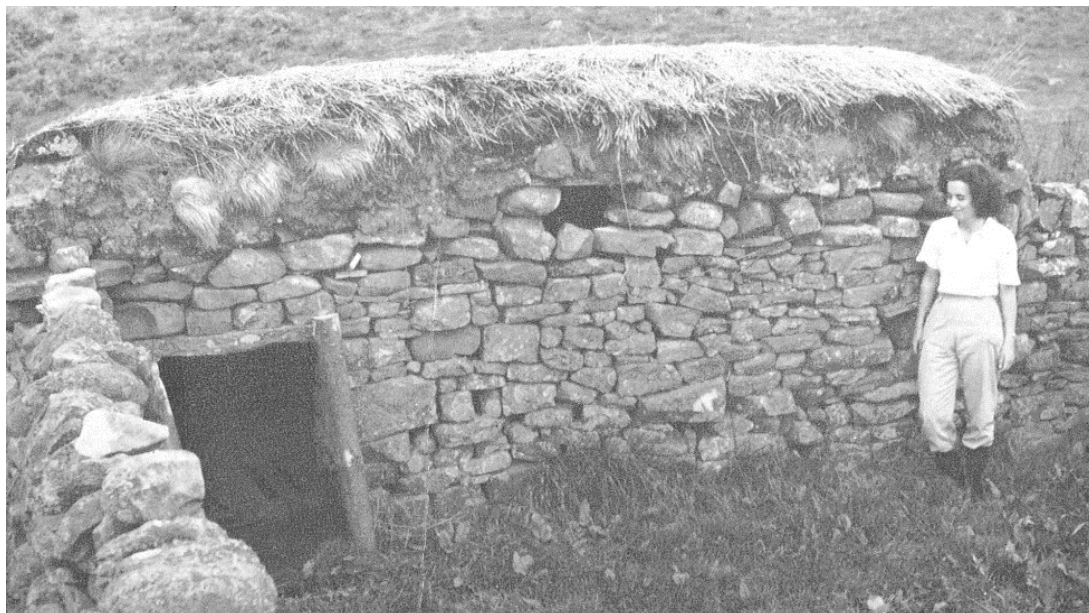
Plate 19: Turf-roofed hut as recorded by RCHME in Northumberland (Ramm et al 1970)
