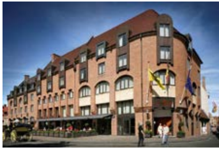
Crowne Plaza Hotel, Bruges: Logis® bath spout, Raindance® 260 Air 1jet overhead shower, Logis® 100 single lever basin mixer, ShowerSelect® thermostats.
