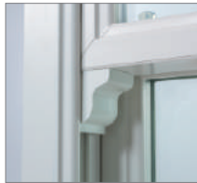
Plant-on Sash Horns
