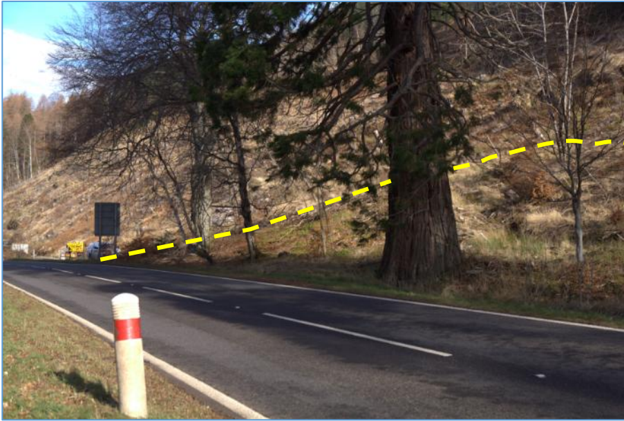
Photo 7: Looking approx. north adjacent to A835. Yellow line shows access route to Mhuilinn powerhouse site using previous harvester track from existing bell-mouth access to construction yard; slope beyond is on north bank of burn.
