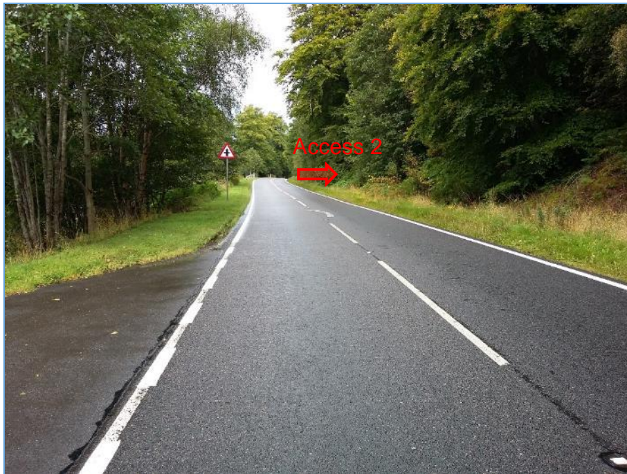
Photo 2: visibility at access 2 is restricted by foliage, sign and bank
