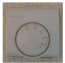
A ROOM THERMOSTAT: controls the overall temperature of your heating system and is usually located in a hall. The room thermostat should be set to the lowest comfortable temperature, typically between 18°C and
