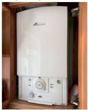
Condensing boilers come in both combination and standard models. A combination (or 'combi') boiler will provide your central heating and produce hot water on demand, firing up when you turn on a hot tap. A standard boiler provides central heating but rather than produce hot water as and when needed, it will heat a quantity of water which is held in a hot water cylinder until required.
