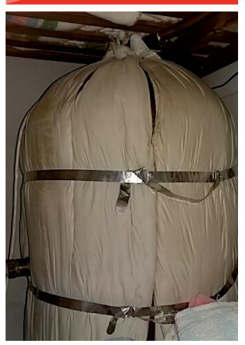
Hot water may come from a tank in your airing cupboard. This should be connected to a timer so that it only comes on when cheaper off-peak electricity is available. If there is not enough hot water during the day, you can press the 'boost' button on the programmer to get more, but this uses expensive on-peak electricity.
