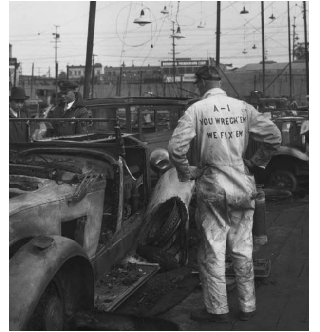
A junkyard worker views burned-out vehicles.
