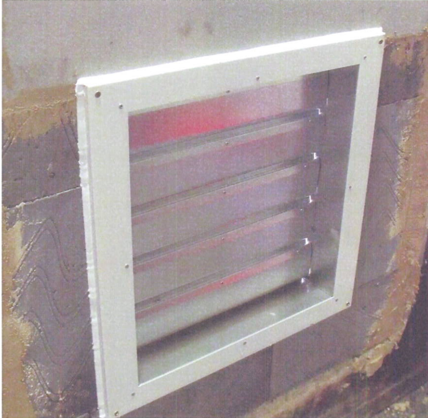
Exposed face prior to testing
