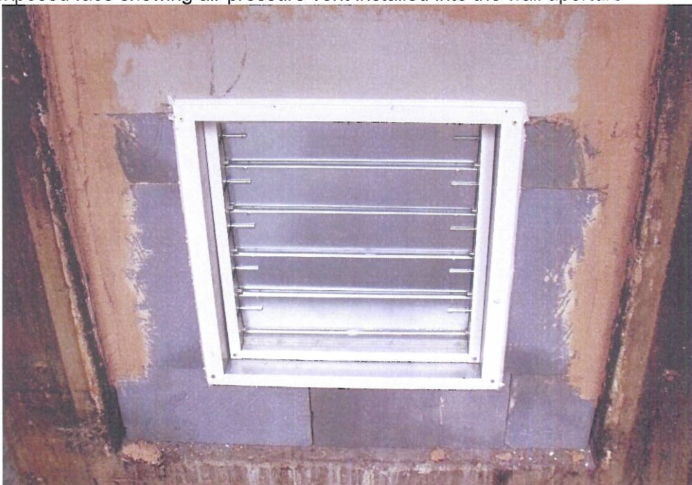
Unexposed face showing air pressure vent installed into the wall aperture
