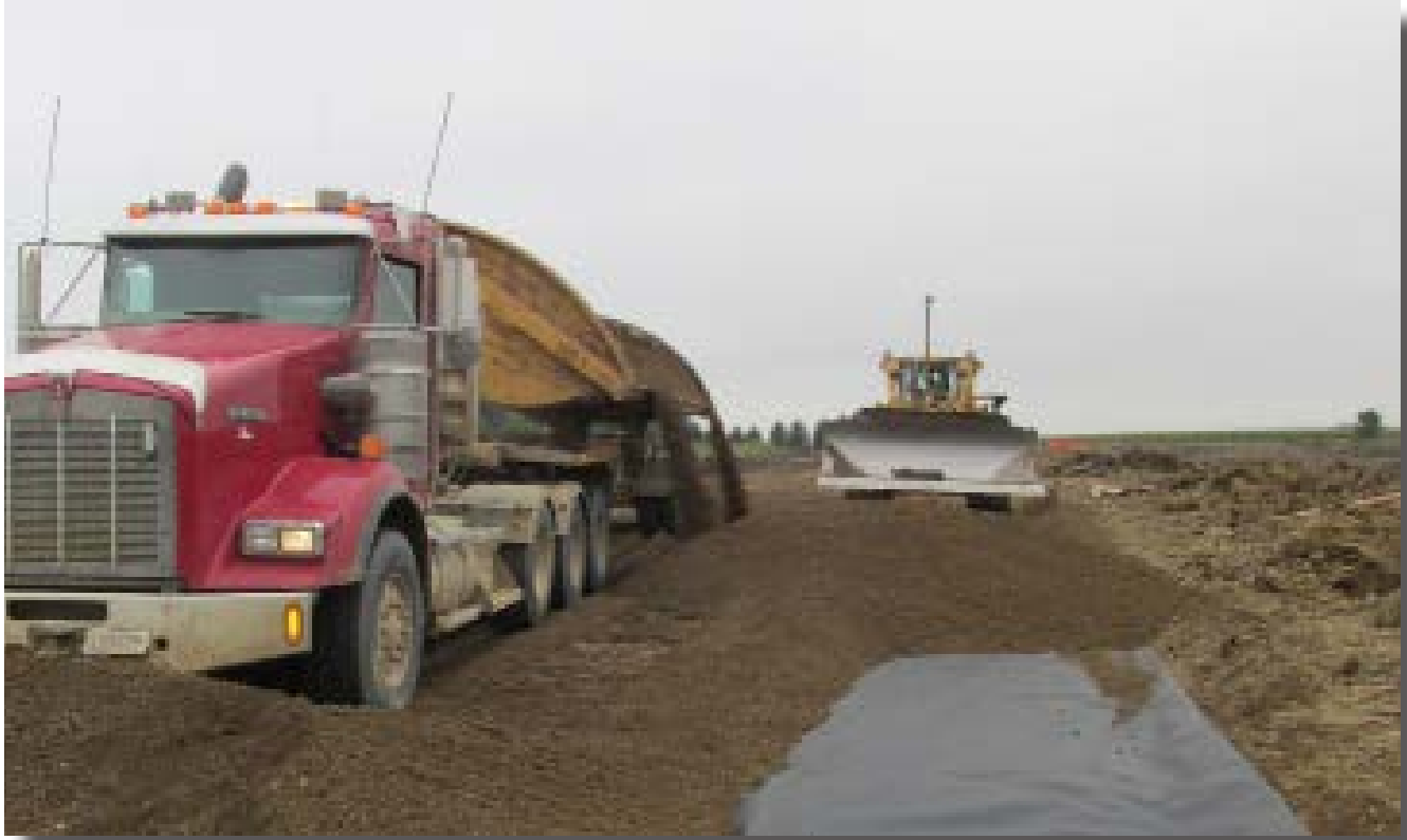
Good practice of dumping and pushing material out over the fabric to avoid damage during construction.
