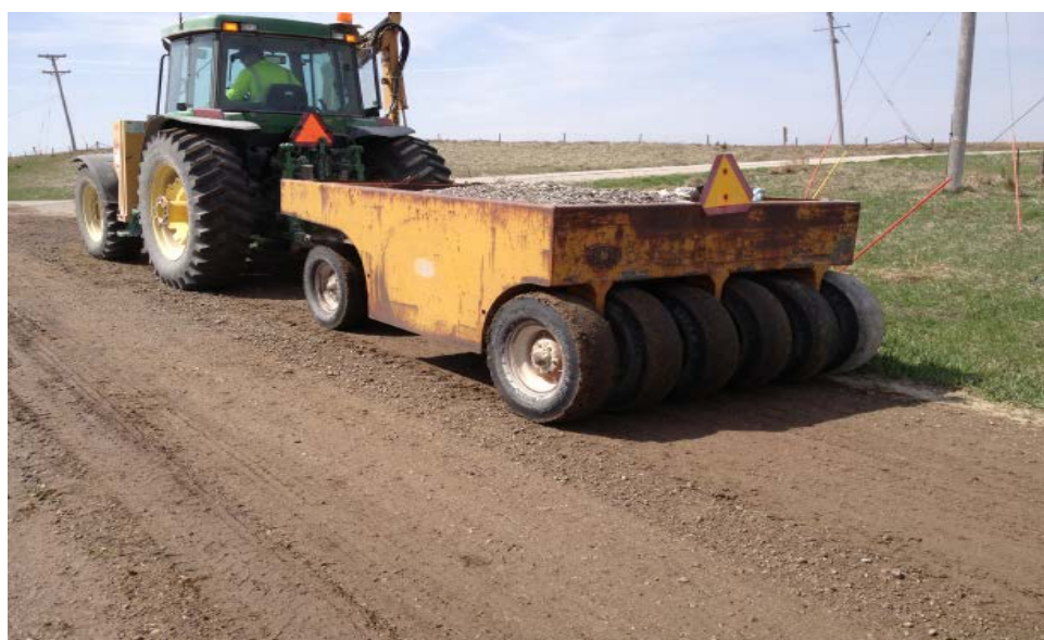
Be careful with premature rolling of chloride treatments when material sticks to the roller and causes an uneven surface. Some agencies do no compaction and have successful chloride treatment projects.
