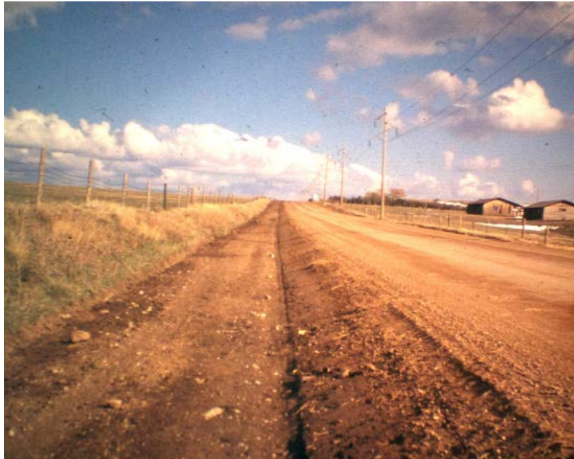
Excellent roadway reshape done with only motor graders, a roller and water truck.
