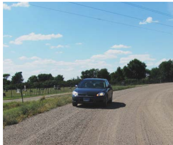
Well-shaped superelevation on a curve.
