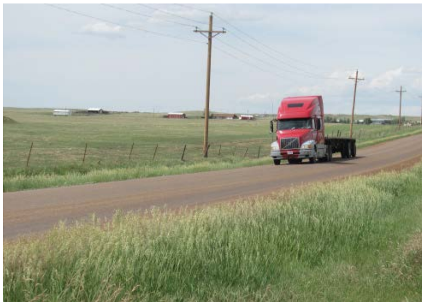
A gravel surface stabilized with liquid magnesium chloride carrying 650 vehicles per day including just over 100 trucks. This is in a semi-arid region.
