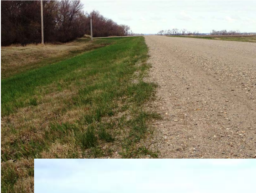
These photos (left and below) show good examples of gravel shoulders that match the edge of the roadway very well and drain water to the ditch.
