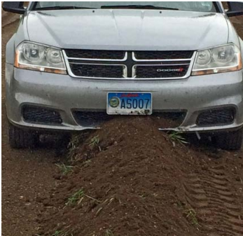
Berm too large for motorists to traverse. (Source: Bruce Drewes, 3T Group LLC).
