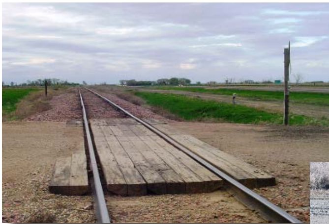
Very well shaped rail crossing on a gravel road.
