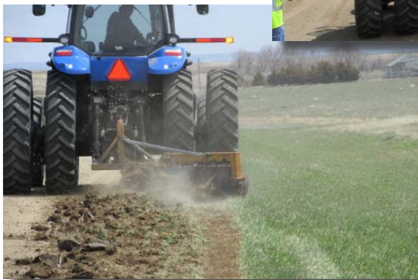
Example of a shouldering disk mounted on a tractor to process sod and gravel before moving it back to the road.
