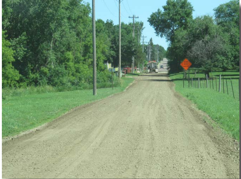
Example of mixed recycled asphalt and surface gravel used on a road with very low traffic.
