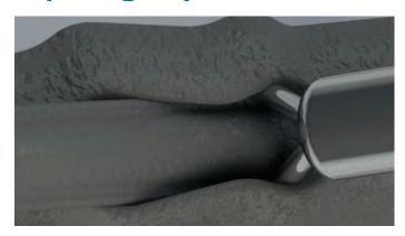
It is now time to fit the filler strip. Before doing this pour a small amount of diluted washing up liquid in the channel that it is to be fitted. Starting at the middle of the bottom, insert the glazing tool into the groove and place the filler strip into the loop of the tool. Run the tool around the groove following the length of filler strip. This should now be placing the filler strip into the groove.
