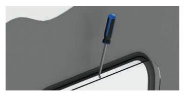
The next step is to remove your window. This can be done by inserting the glazing tool into the top middle face of the seal and pushing around the back of the window. The window can then be levered forward towards you and lifted away. The old seal can now be removed.
