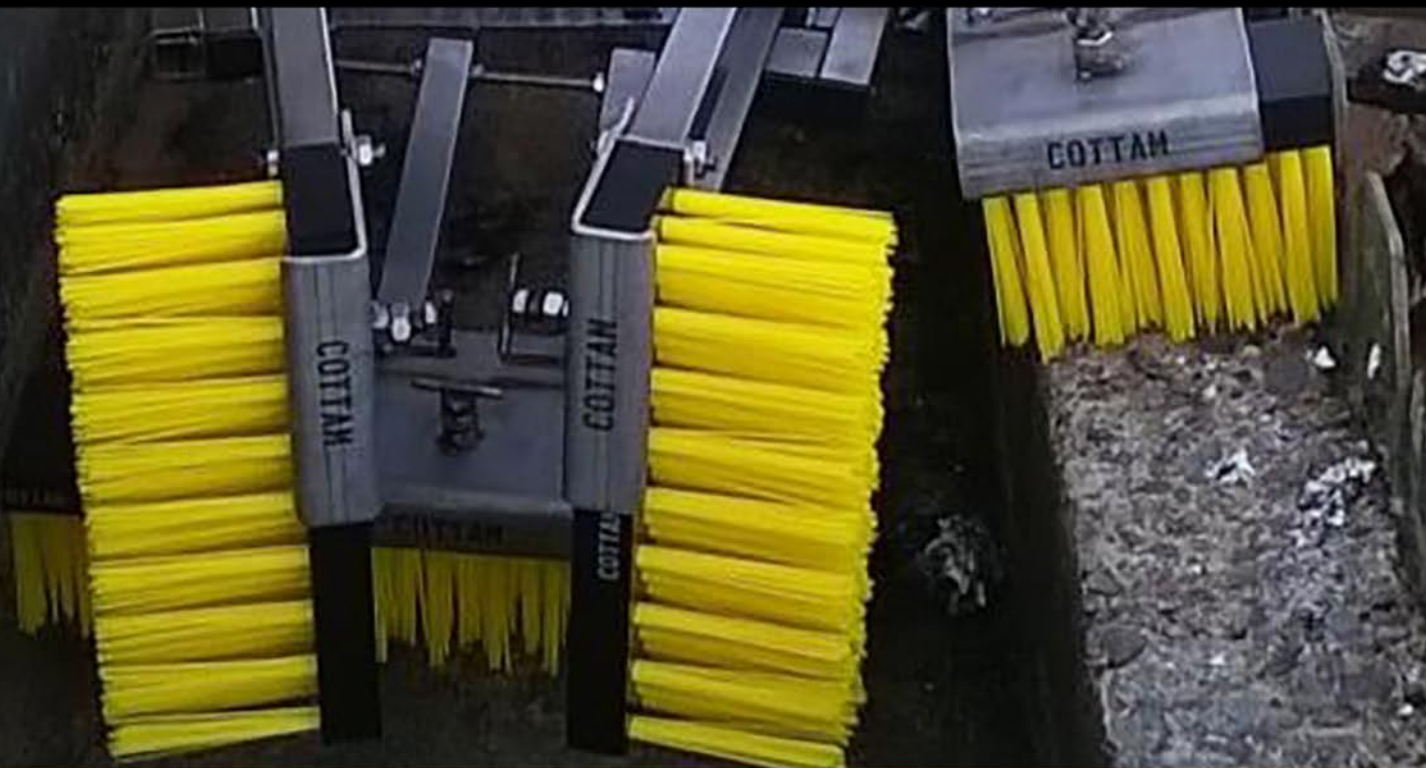
Water Treatment Weir Brushes
