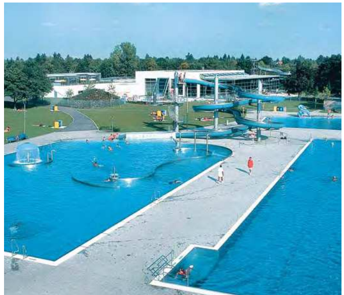
Figure 8: This swimming pool in Munich, Germany was relined with Type 316 stainless steel panels that were welded together. Photo courtesy of Martina Helzel
