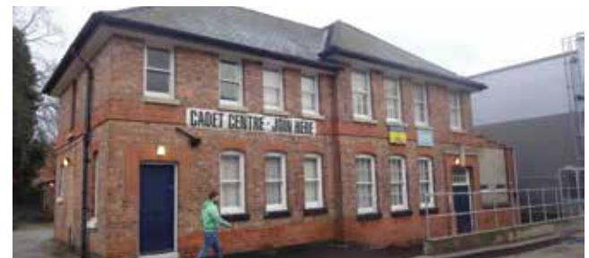
The existing Hinckley Cadet Centre building
