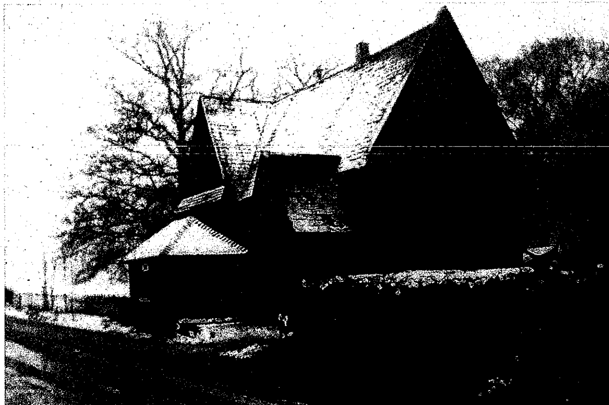
Old school house at Croft: Yes, we were staying here in this weather. No, there wasn't any heating. © Neil Edwards
