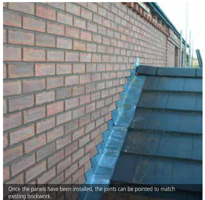
Specially designed panel overlaps ensure a durable and weatherproof finish.
