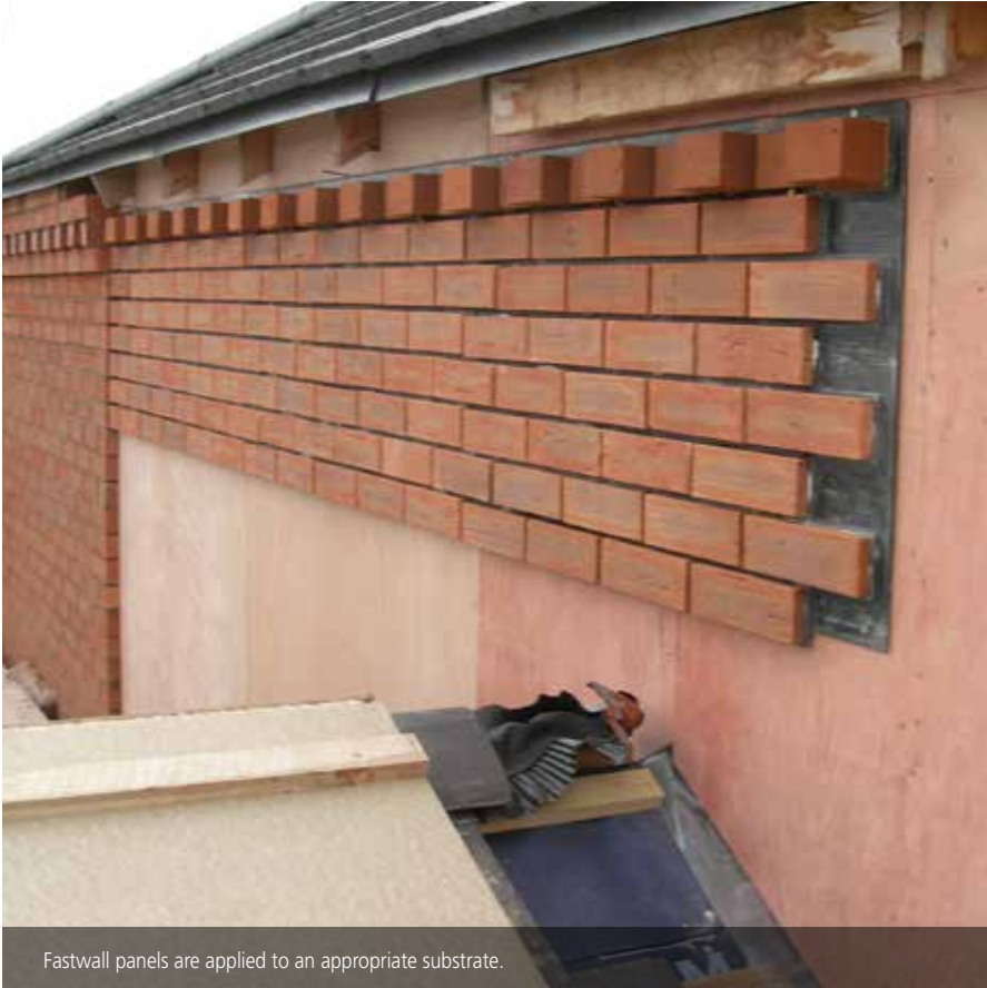
The panels are aligned with the existing brickwork and secured through the fixing points provided.
