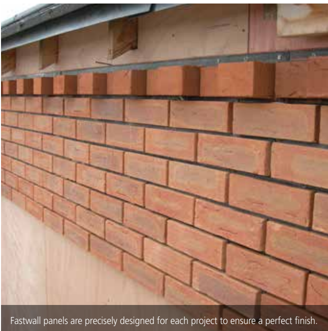
Fastwall panels are applied to an appropriate substrate.
