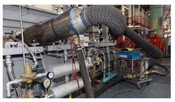
Finally the service division of HORN **heats up** the furnace to operation temperature with special heat-up burners and measurement equipment to ensure the proper temperature gradient and controlled expansion of all refractory material.
